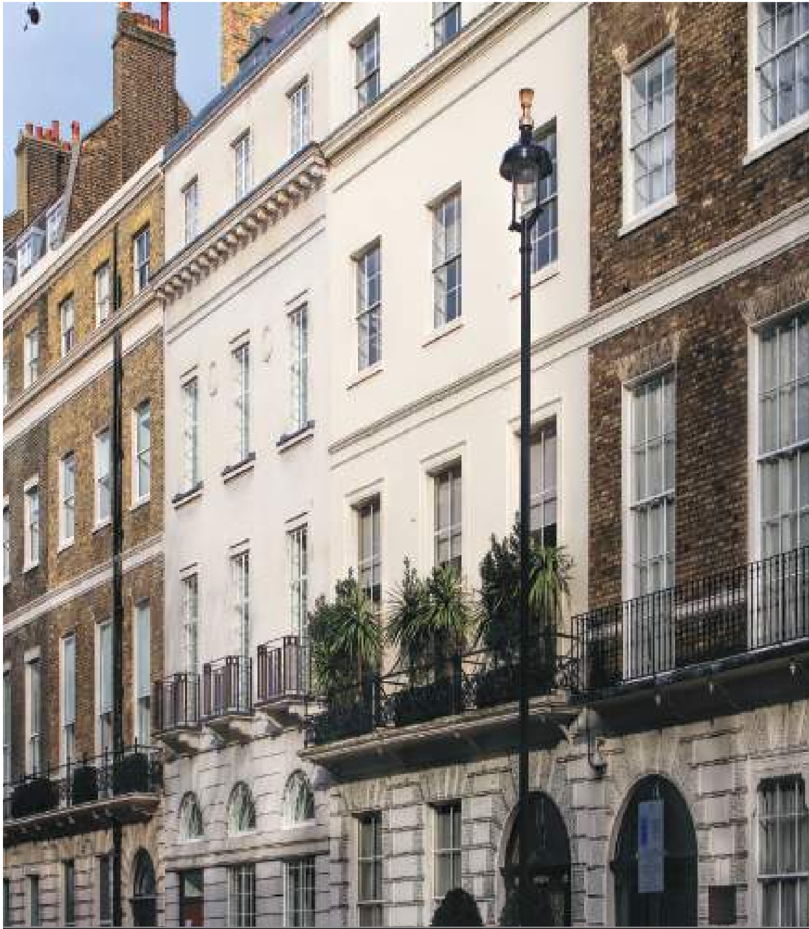
54 PORTLAND PLACE Complete lighting Turnkey to all areas. Private Apartments and Landlord Areas.
