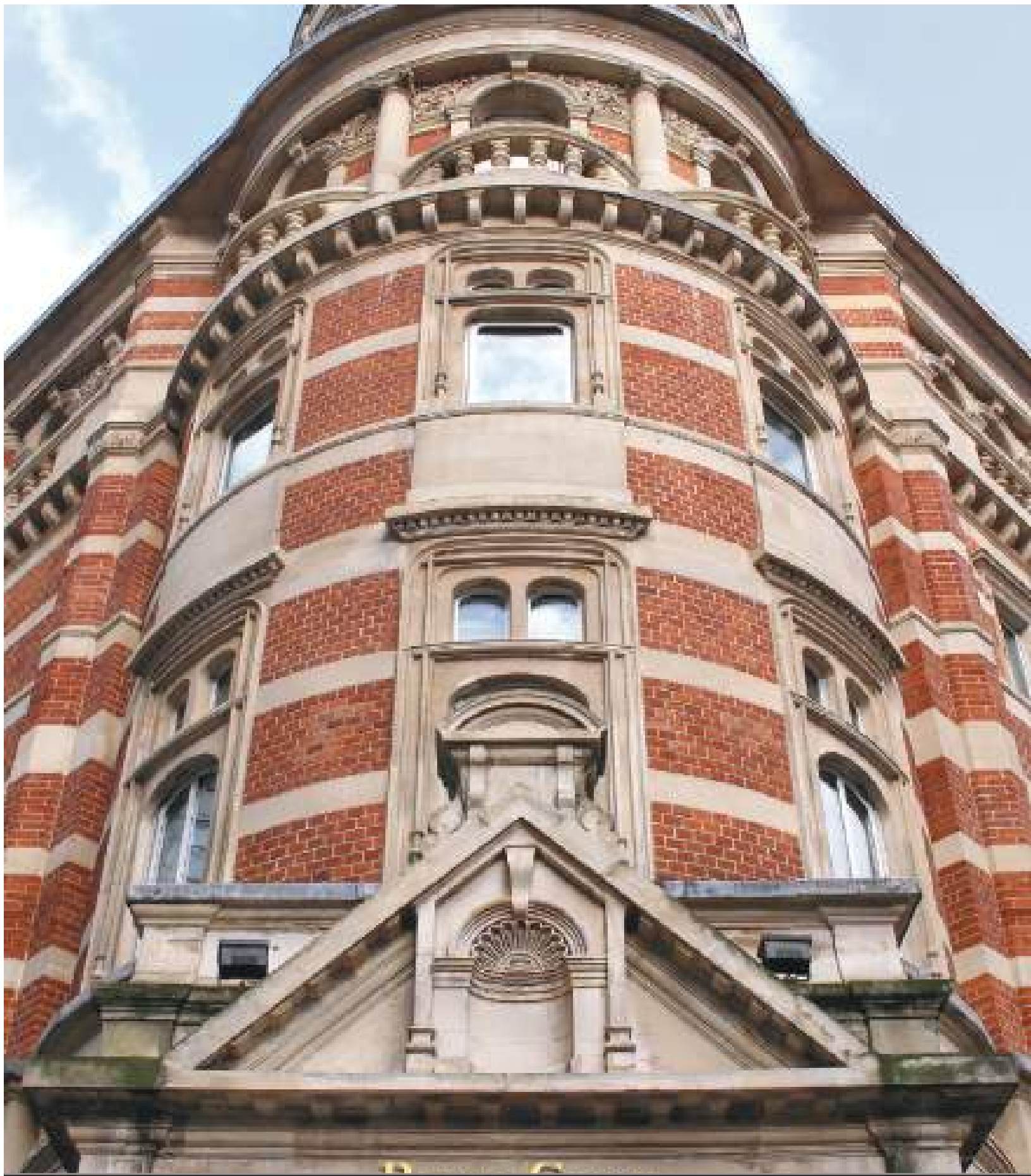
RYDER COURT Commercial lighting fitout. Offices, Front of House, Back of House and Welcome Areas.
